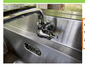
Attach the faucet fittings when using, and remove and store after use.
